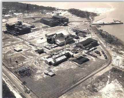
Ethyl-Dow Plant Bromine Extraction at Kure Beach, NC (Photo from NC DNCR)
