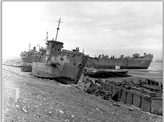
Photo SC 193919 Broached LCI(L)-92 and other landing craft on Omaha Beach during storm 21 June 1944.
